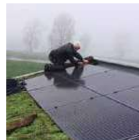
PV-panelen / zonneboiler / ect.
